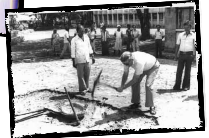
Fr RW Norman, SJ, at the groundbreaking ceremony of Neelima Acharji Hostel
